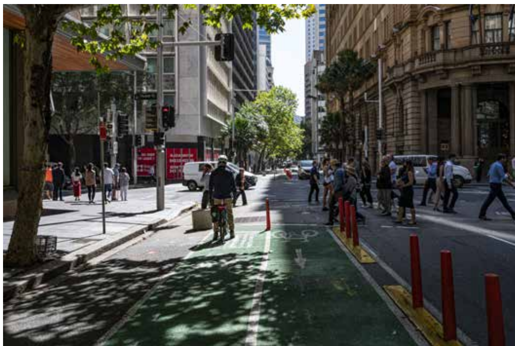
Pitt Street - temporary cycleway
